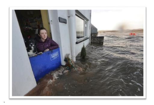
Although there are lots of different types of gates, what most have in common is that they rely on a rubber, foam, sealant or neoprene seals - so think ahead. These products usually get stored in a garage or shed and may not be used for a number of months, but all seals will over time deteriorate, get knocked or may even get a nibble from a mouse. Be sure to get a clear understanding from the supplier so that you know
