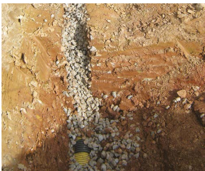
Figure 37. Washed gravel permeable fill over drain
