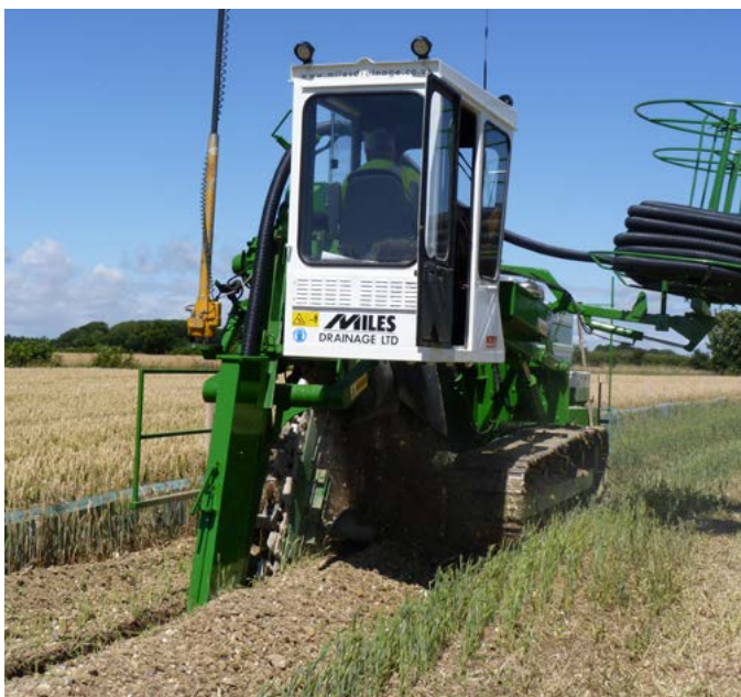
Figure 31. Installing land drains with laser gradient control
