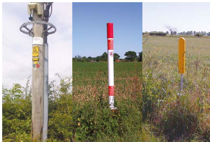
Figure 18. Signs indicating potential underground hazards
