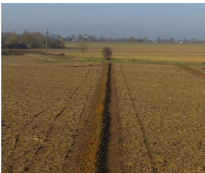
Figure 29. Recently installed drains
