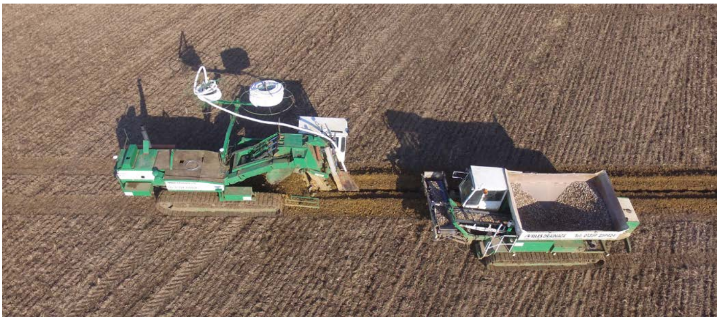
Figure 28. Installing land drains and stone backfill
