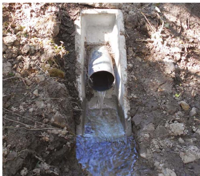
Figure 38. Precast concrete headwall (type K)
