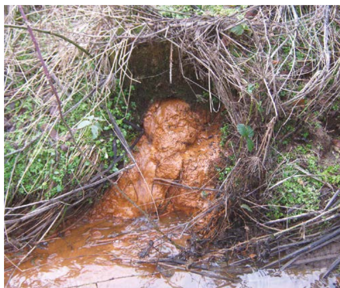
Figure 24. Drainage outfall blocked by ochre
