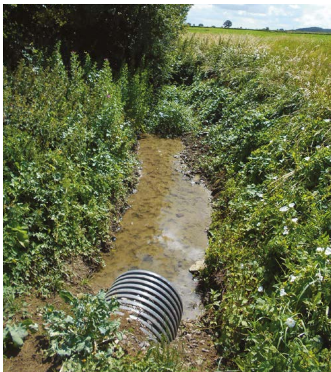
Figure 20. Cleaning ditches is a simple way of improving the effectiveness of drainage systems
