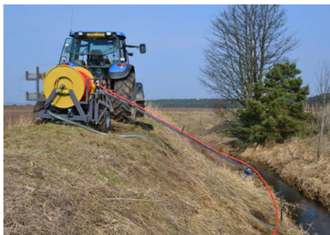
Figure 23. Drain jetting
