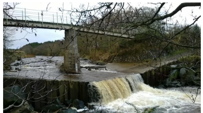
The existing major weir and footbridge at Haugh Head
