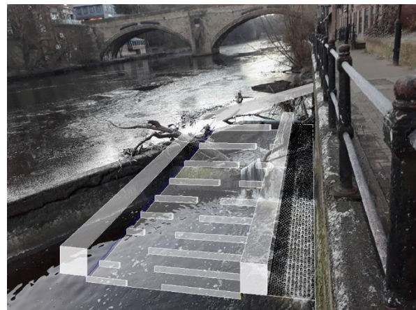
Visualisation of a low cost baffles fish pass for Framwellgate upper weir
