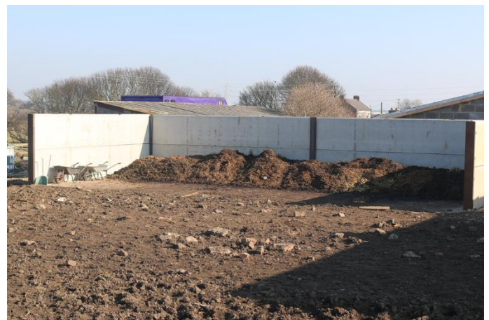
Before and after improvements to muck storage facilities
