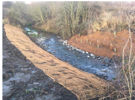
Before and after erosion repairs
