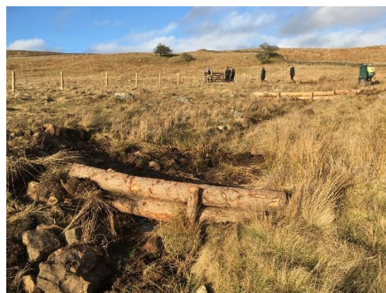
A series of high flow deflectors will reduce sediment
