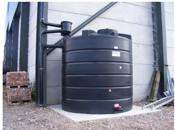
Rainwater harvesting on farm to reduce surface water runoff and diffuse pollution
